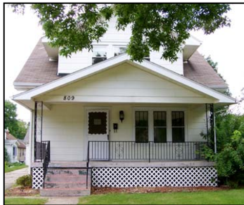
Figure 2.5. Vacant Home in Good Condition, Summer 2008
