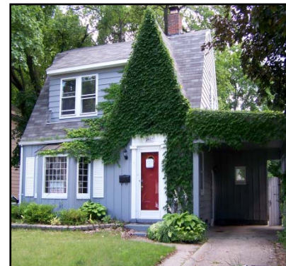
Top: North-Northeast Zone, fair condition Center: Central Transition Zone, poor condition Bottom: South-Southwest Zone, good condition
