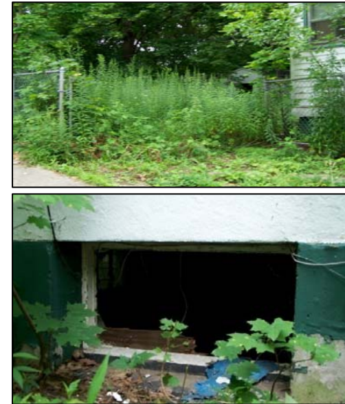
Figure 6.5. Photos of Code Violations, Summer 2008
